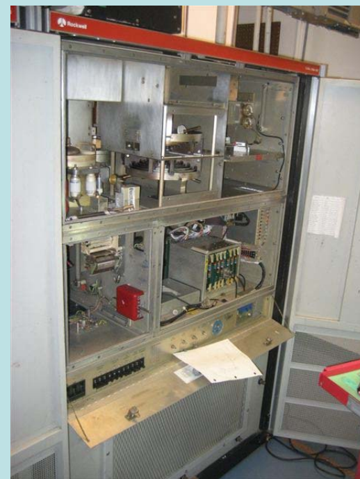
Rockwell Collins 10KW HF80 transmitter - at end of useful life
